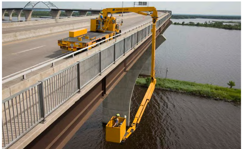
Figure 2.5.20 Under Bridge Inspection Vehicle with Bucket
