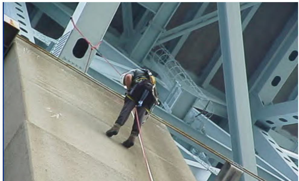
Figure 2.5.9 Inspector Rappelling Substructure Unit
