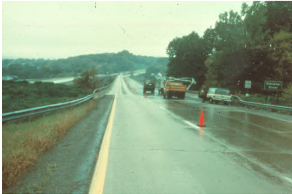
Figure 2.2.12 Inclement Weather Causing Slippery Bridge Members and Poor Visibility for Motorists
