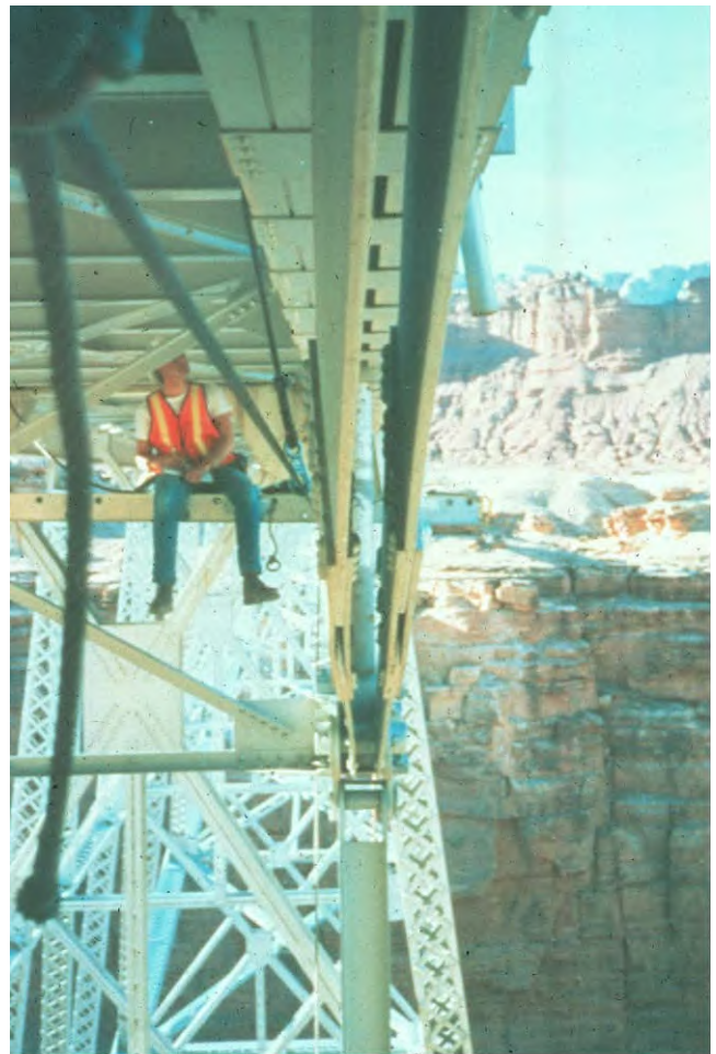
Figure 2.5.4 Rigging for Superstructure Inspection
