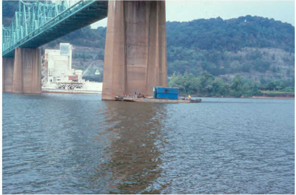
Figure 2.5.6 Inspection Operations from a Barge
