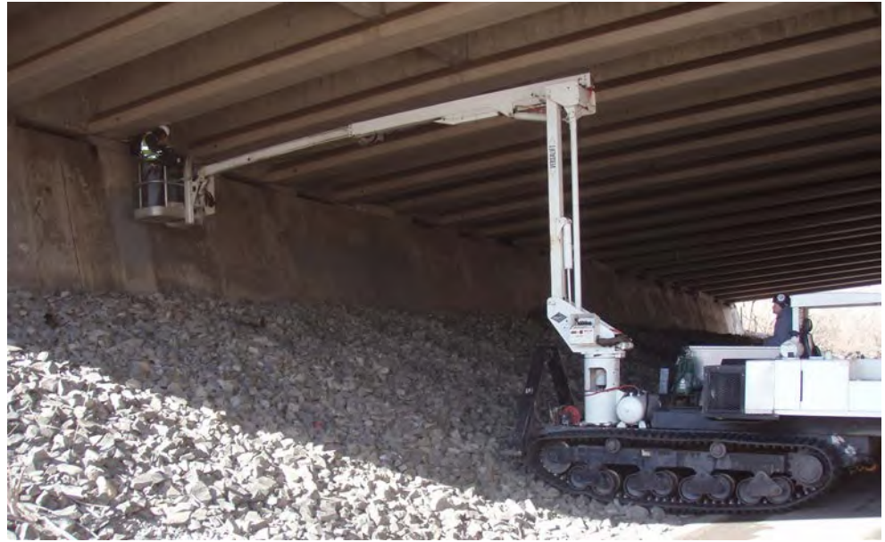
Figure 2.5.19 Track-mounted Man-lift on a Slope
