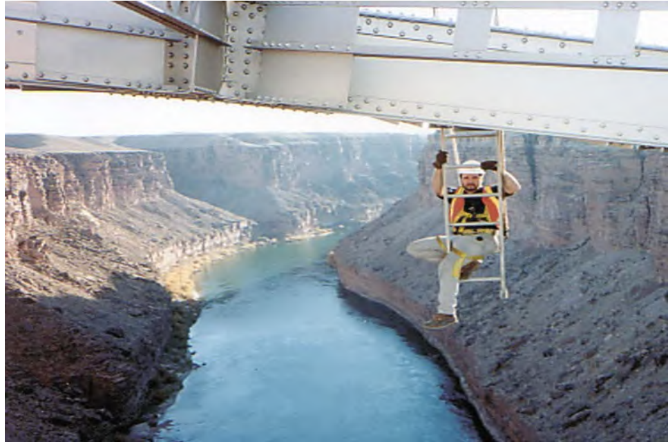
Figure 2.5.2 Inspector using a Hook-ladder
