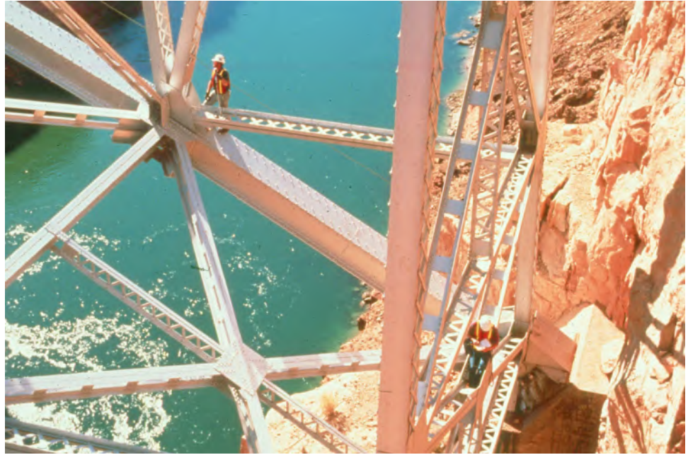
Figure 2.2.7 Inspection Involving Extensive Climbing
