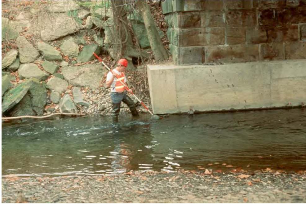
Figure 2.1.5 Inspection for Scour and Undermining
