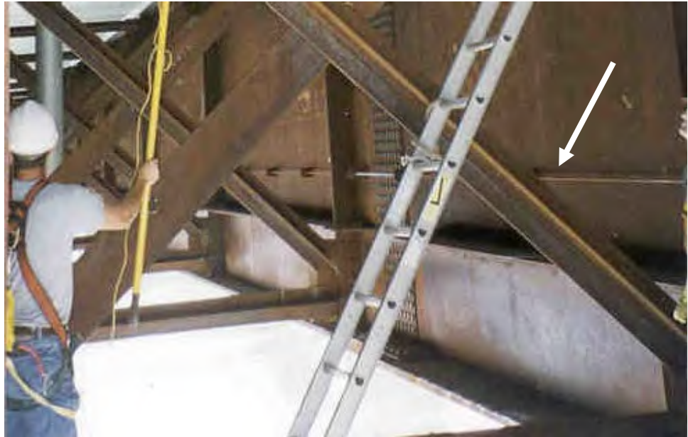
Figure 2.5.13 Handrail on Girder Bridge
