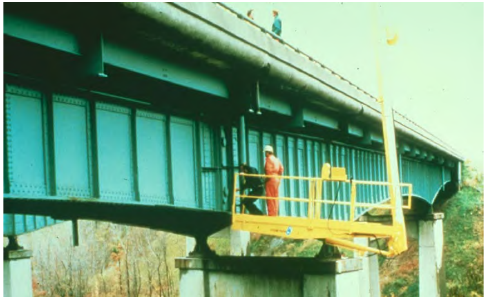
Figure 2.5.21 Under Bridge Inspection Vehicle with Platform
