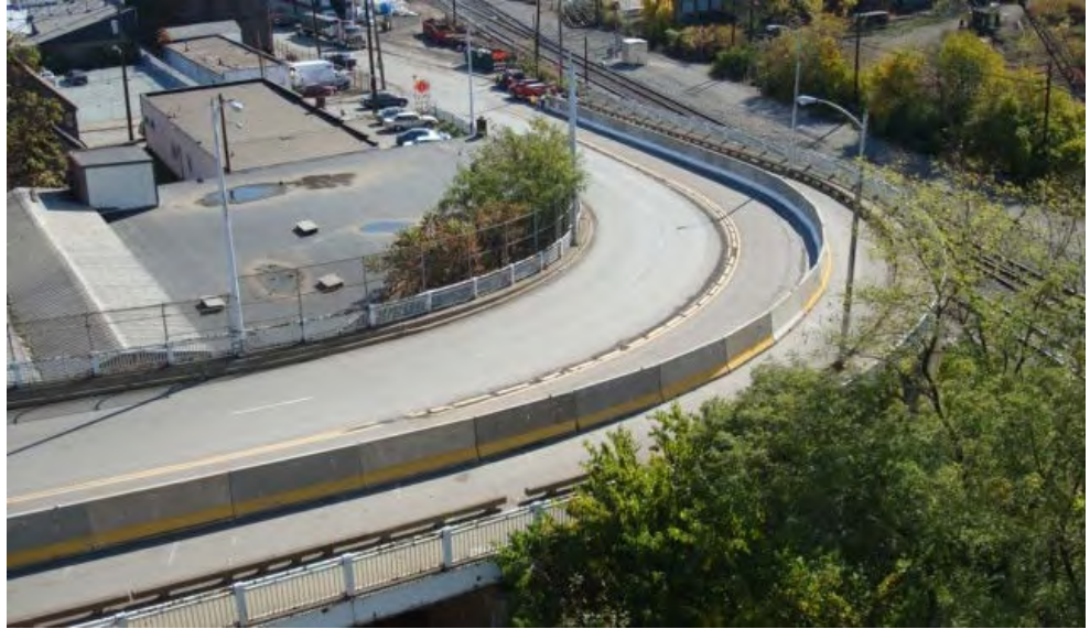
Figure 2.3.13 Temporary Traffic Barriers
