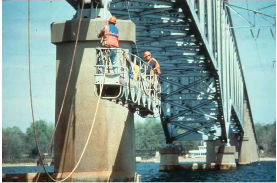
Figure 2.5.3 Rigging for Substructure Inspection
