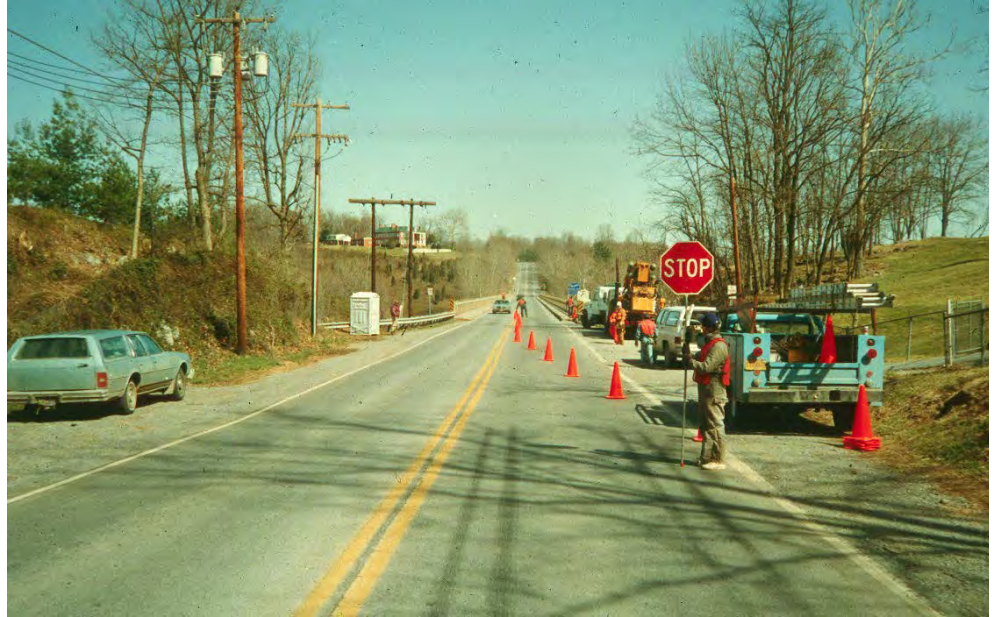
Figure 2.1.4 Temporary Traffic Control Operation
