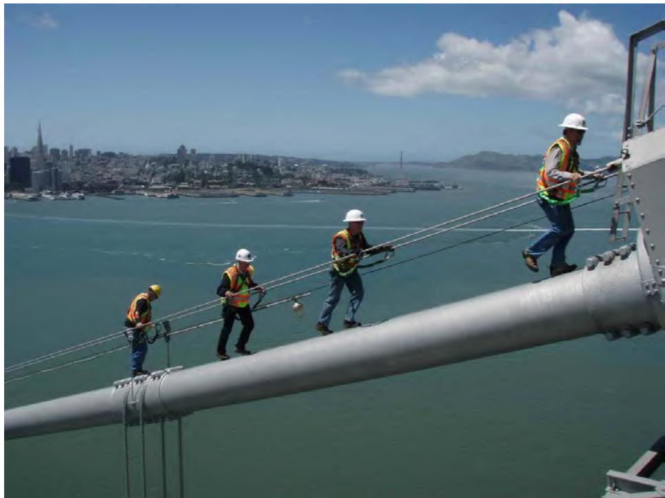
Figure 2.5.14 Handrail on Suspension Bridge
